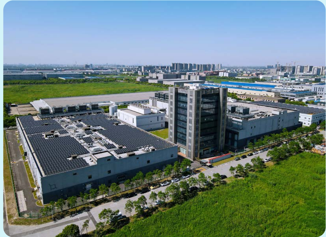
Rooftop solar at SH1, Shanghai Campus
