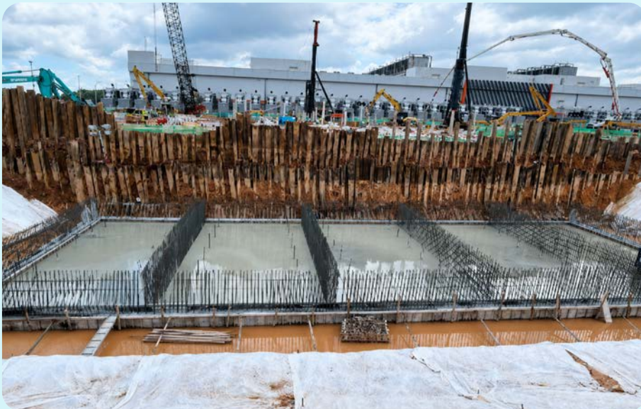
Application of Code+ 505 and Code+ 515 at Fuel Tank Area
