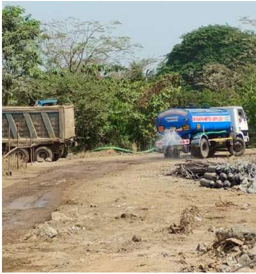
Access Road with Dust Suppression
