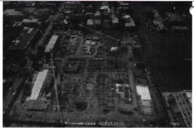
Fig: Construction at the site
